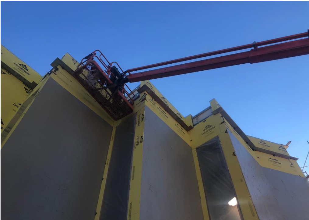
Sheathing Progress at West Elevation
