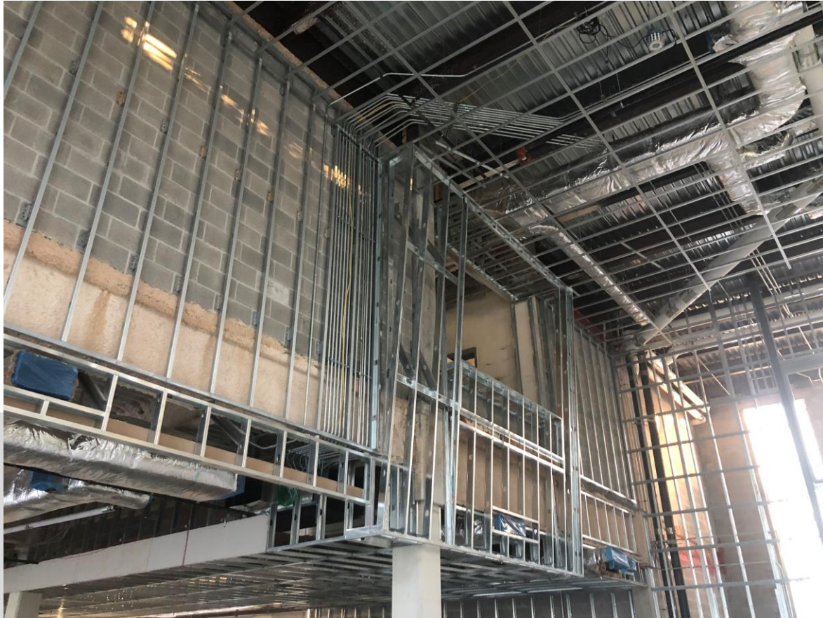
Metal Framing Progress in New Addition Media Center
